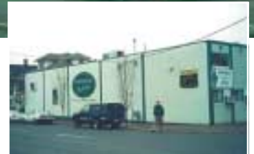
Quimby Retail Building, before.
