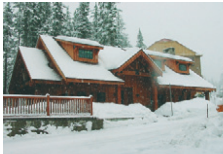
The Collins Lake Club House, completed in time for winter, provides a cozy recreation facility for the resort and includes an outdoor pool and spa.
