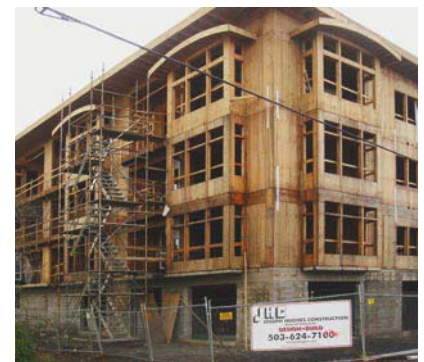
Right: Twelve condominium units on top of structured parking reach for the sky in Seaside, Oregon, as framing is completed at Riverside West Condominiums. This project, designed by Tom Johnson, Architect, of Portland, and developed by RSWC, LLC, will be ready for occupancy later this year.
