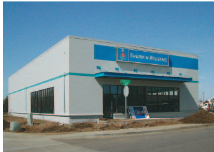
This 5,000-square-foot concrete block building was designed by RAR Architects and developed by Hunt Leigh Development Vancouver LLC. It is the new location for Sherwin-Williams in Vancouver, Washington.
