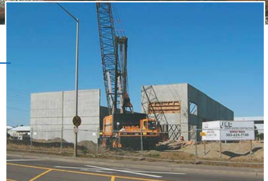
Chin's Import/Export coming out of the ground in these September photos. JHC Commercial, LLC teamed with the owner, Keith Lee, and CIDA Architecture & Engineering on this 20,000-square-foot design-build tilt-up concrete building.
